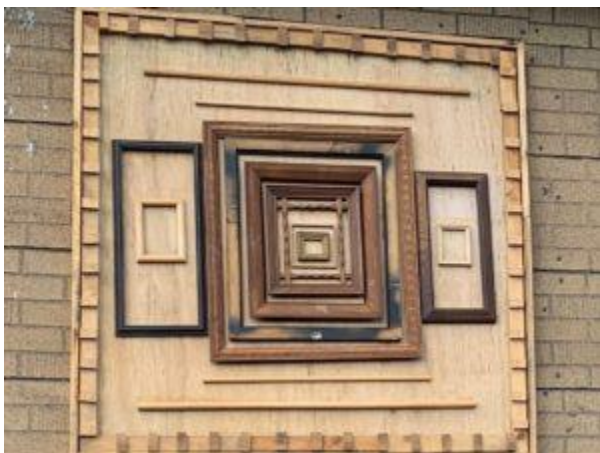
#18-16, Log Cabin Windows 4562 Highway 88 Pine Ridge AR
